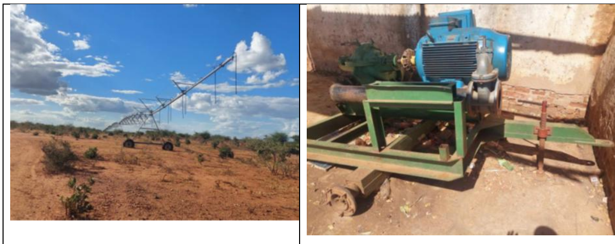
Plate 5: Facilities at Chiwirirano Irrigation Scheme
