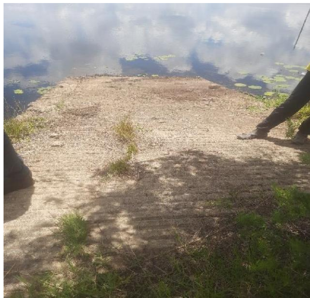
Plate 1: Pump Ramps at Don Rungano Irrigation Scheme
